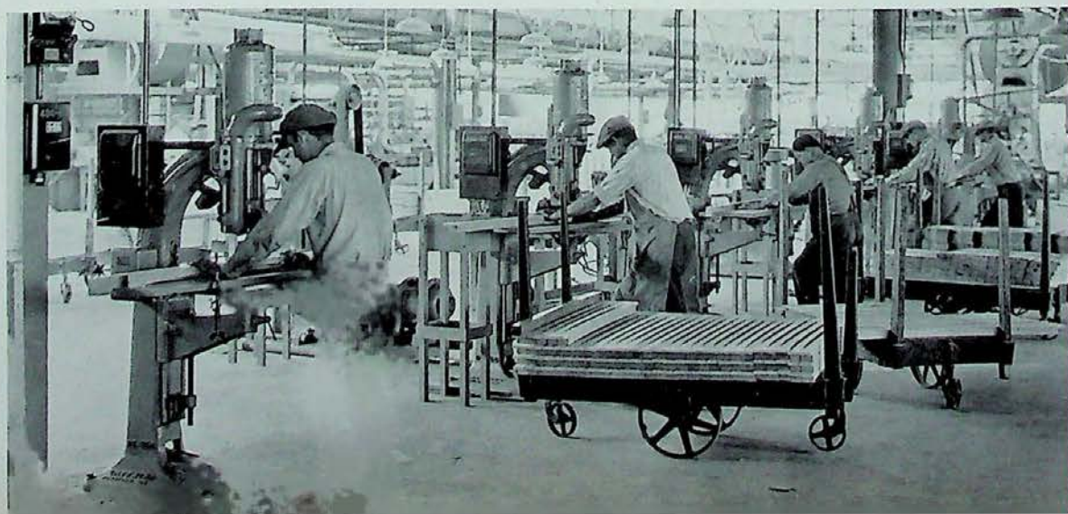
Five Greenlee No. 356 Single-Spindle Borers in a Modern Industrial Plant
