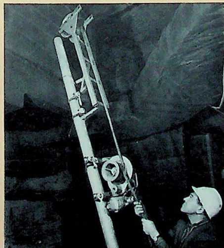
Setup for horizontal pull from a ceiling-mounted pull box, using 640 power puller and 649 pipe adapter sheave. Built-in chain clamp mount units rigidly to pulling boom improvised from piece of 3" galvanized conduit.
