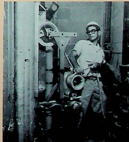
Compact design of Greenlee cable pulling system lets you make tough pulls in tight spaces too small for other pullers. Here Nos. 649 sheave and 640 power puller are set up for an "up" pull in a cramped closet.
